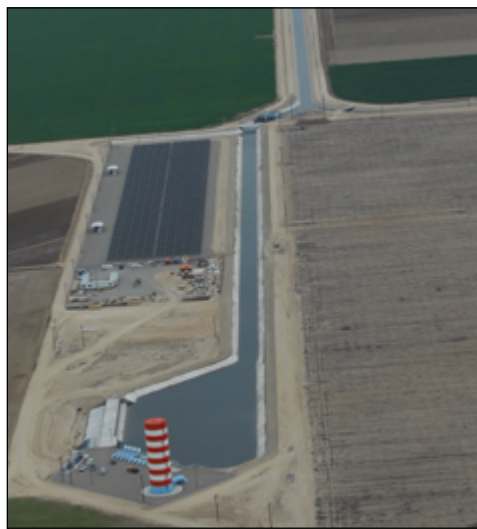
Semitropic Junction pumping plant — west of Wasco, California — where both ground and surface water can be redirected according to water banking agreements between the agricultural district and urban water districts north and south. Photo courtesy Semitropic Water Storage District.
