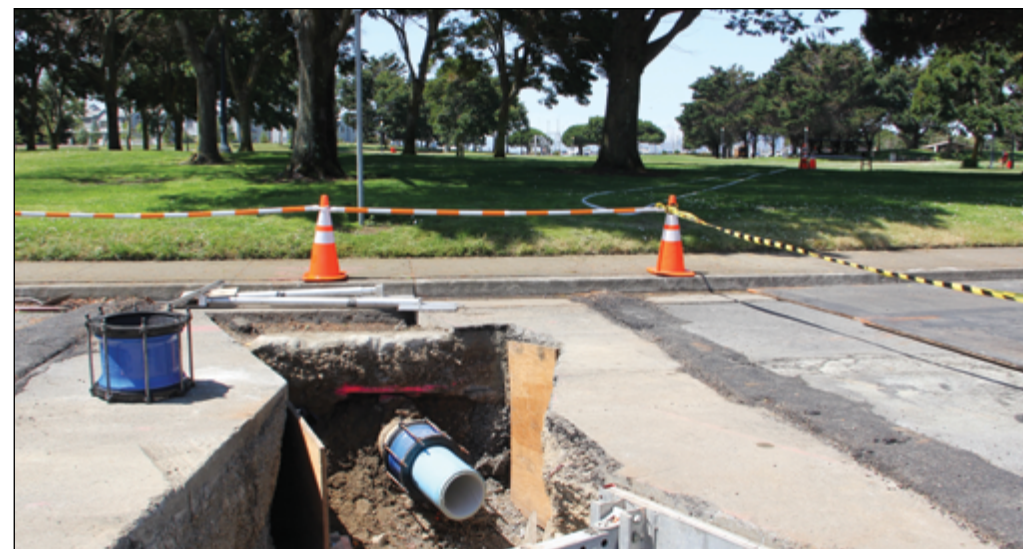
Marina Park in Richmond, where installation of Aqua-Pipe avoided the disruption to park services of extensive trenching. Photo: EBMUD
