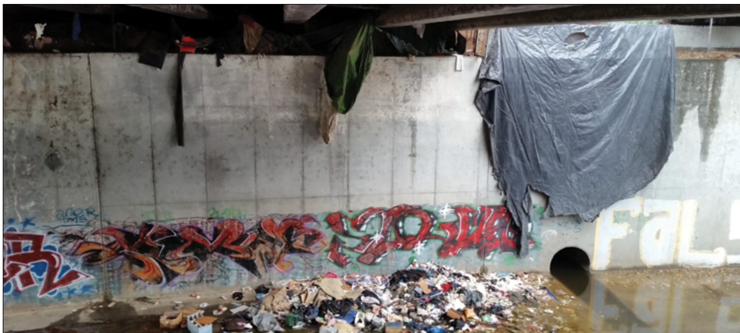
Trash in Walnut Creek and stormwater channel. Photo courtesy Contra Costa Flood Control and Water Conservation District.
