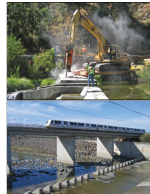
In 2006 the San Francisco PUC removed Sunol and Niles (pictured) dams from Alameda Creek, alleviating public safety concerns and providing steelhead and other fishes' access to upstream waters. The flood control channel downstream (BART photo) still presents various obstacles to fish. Photos by Brian Sak.
