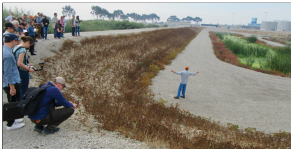
Participants in Resilient by Design challenge stand at the top of horizontal levee looking over an associated wet weather basin, with the jungle of growth on the new levee behind them.
