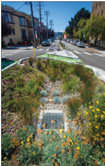
Rain garden in San Francisco's Mission District funded by an SFPUC green bond. In November 2018, Los Angeles County approved another innovative financing mechanism: Measure W. Starting in 2019, property owners will pay 2.5 cents for each square foot of impermeable surface on their parcels. The tax will raise an estimated $300 million per year to fund rain gardens, parks, and watershed restoration designed to capture and clean the precious rainwater running off the county's concrete and asphalt surfaces. Photo: SFPUC
