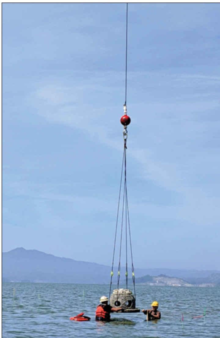
Triton Marine lowers a reef ball from crane. Photo: Avra Heller
