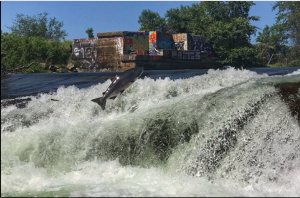
Spring run Chinook passing over Durham Mutual Springer Dam. Photo: Scott McReynolds
