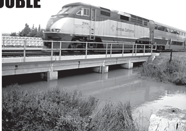
The waters of Pinole Creek rise beneath this new railroad trestle during a January storm and five-foot tide. The storm was probably only a "two-year" event. Photo courtesy of Carol Arnold, Friends of Pinole Creek.
