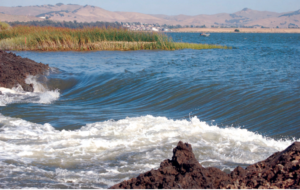
Salinity reduction breach in the South Unit of the Napa Plant Site Restoration Project opened to tidal action for the first time in over 100 years on August 25, 2010. The plant site was previously used for solar salt production. Due to residual salt issues, breaching events were carefully phased to minimize the potential for adverse water quality conditions to the Napa River. Photo courtesy Karen Taylor, CDFG.
