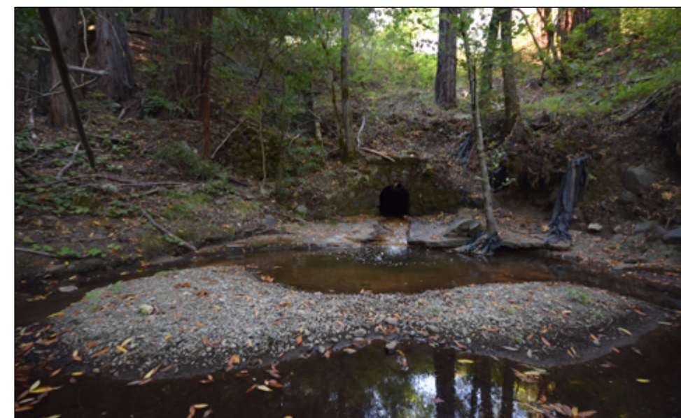
Dam outfall before removal. Photo: California Water Audit
