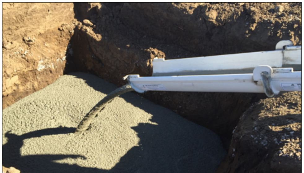
Backfilling the new sewer trench with a lean concrete slurry, which is stronger and less expensive than backfilling and compacting with soil. Photo: Sonoma Water
