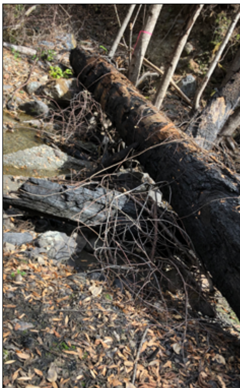
Log sediment structure anchored to tree. Photo: Daniel McGlynn
