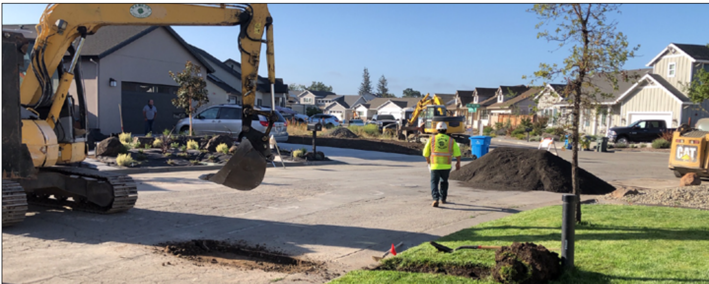
Connecting a sewer lateral. In some parts of the Larkfield project, contractors used a technique called trenchless installation to save cost. The technique involves drilling a small tunnel and pulling a long high-density polyethylene hose/pipe behind it. The driller aims the tunnel to a pit several hundred feet away where they connect to a conventional sewer pipe. Photo: Sonoma Water
