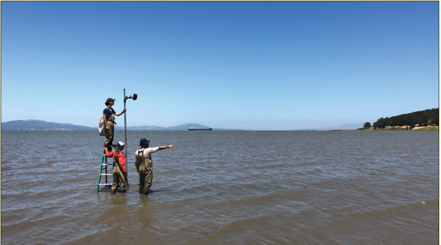
ESA field staff orient and install a time-lapse camera at the Giant Marsh project site, in order to document wave run-up along the marsh shoreline. Photo: ESA
