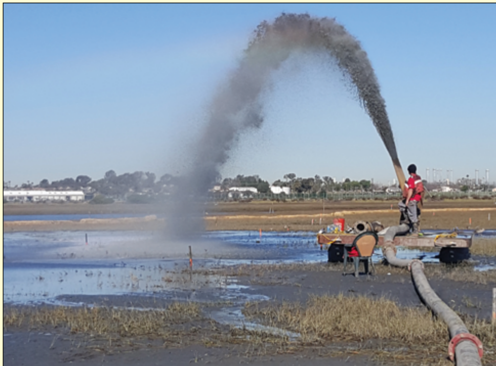
Nozzle used to apply sediment at Seal Beach (note the one pictured is elliptical as recommended for future applications). Photo courtesy USFWS.
