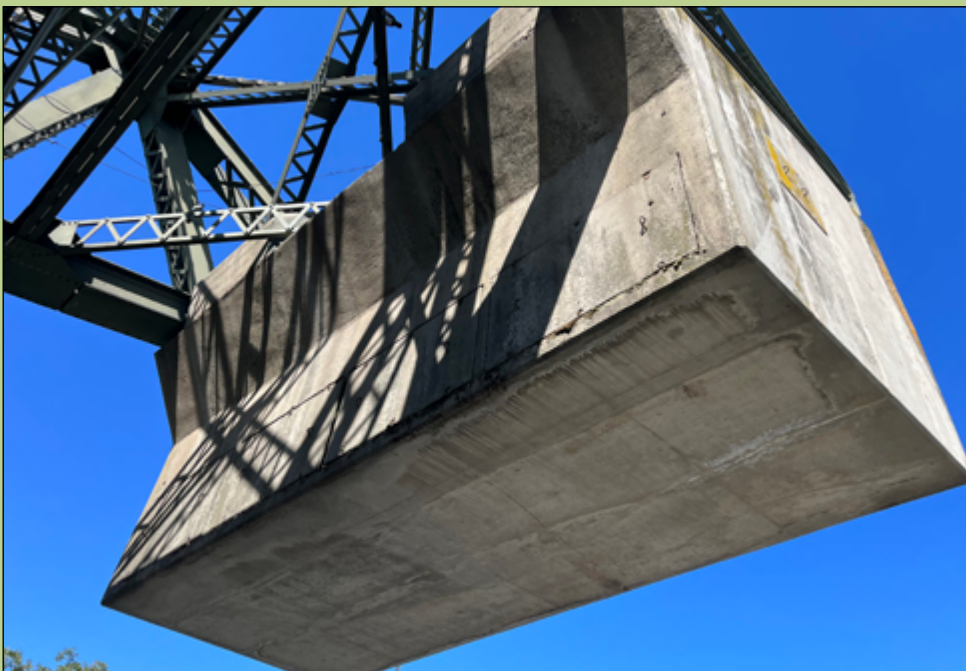
Bridge counterweight. Photo: Aleta George
