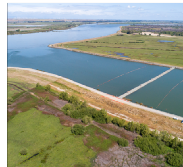
West False River Barrier, looking northwest, near the confluence with the San Joaquin River. Photo: Florence Low, DWR
