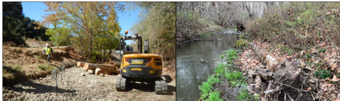
LEFT: Placing spawning gravels on top of creek bottom to improve fish habitat, Los Gatos Creek, 2019. Photo: Valley Water. RIGHT: Woody materials attached to bank by cables, Feb. 2022. Photo: Baykeeper.
