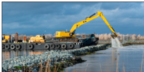
Crews make a notch in the drought barrier in January 2022 to allow fish and vessels to pass through. Photo: DWR
