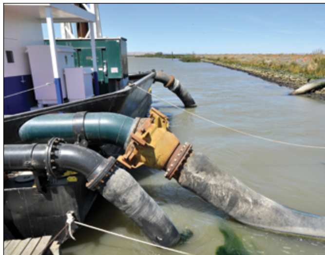
Techniques used to add sediment to the Montezuma Wetlands included hosing it from a sediment laden barge. Photo: Darren Graffius
