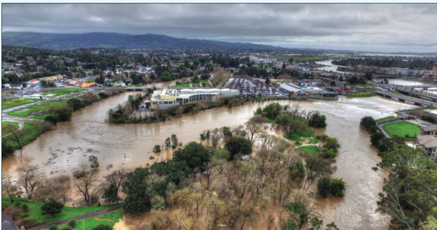
One of the most ambitious and successful flood control projects in the region to date created much more space for water to spread out from the Napa River. The project has performed admirably in subsequent storms, including recent deluges like the one pictured here in 2017. Photo: Napa RCD
