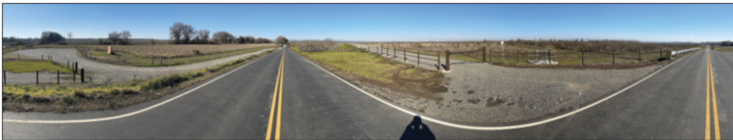
A view of the new setback levee from Road 23. Photo by Daniel McGlynn
