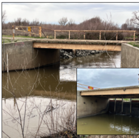
Los Rios Check Dam open for fish passage and with boards blocking passage (inset). Photos: Max Stevenson.
