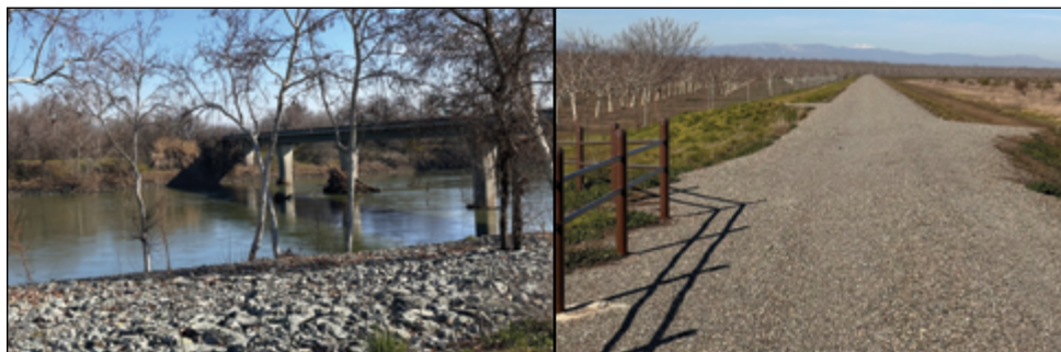
The north side of the Highway 32 bridge right outside of Hamilton City. The bank near the bridge footing is protected by rock. Photo Daniel McGlynn
